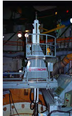
Mast-type remote handling machine
