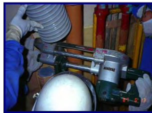
Cutting of pipe by rotary band saw
