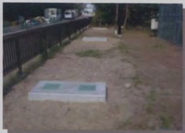
Foundation for pipes
