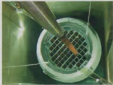
Fuel Loading in Fuel Pool
