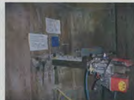
Concrete core Bowling of biological shield wall
