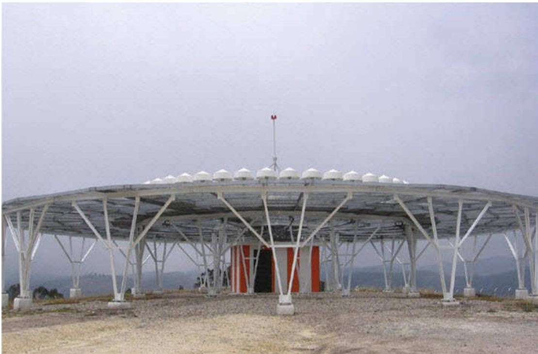
Figure 1-2 Dual Doppler VHF Omni-range (DVOR) Station with DME
