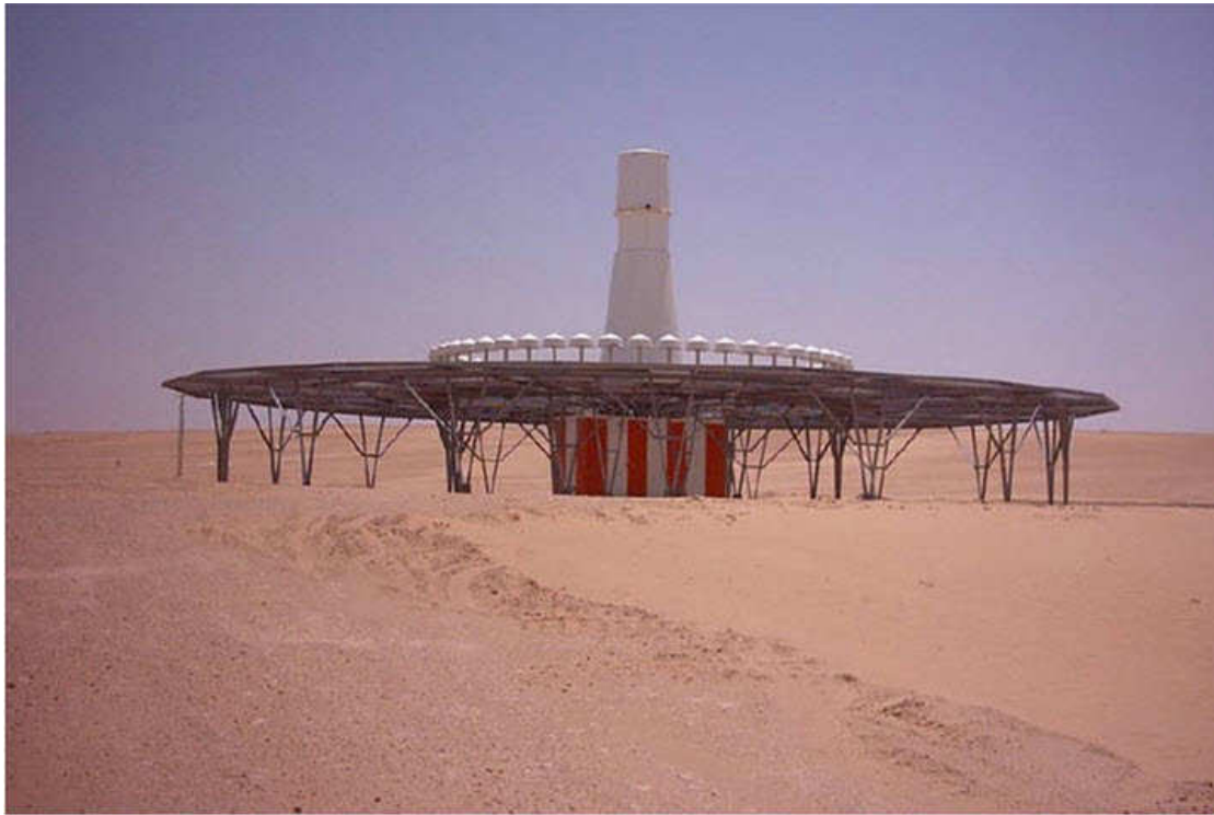
Figure 1-1 Dual Doppler VHF Omni-range (DVOR) Station with TACAN
