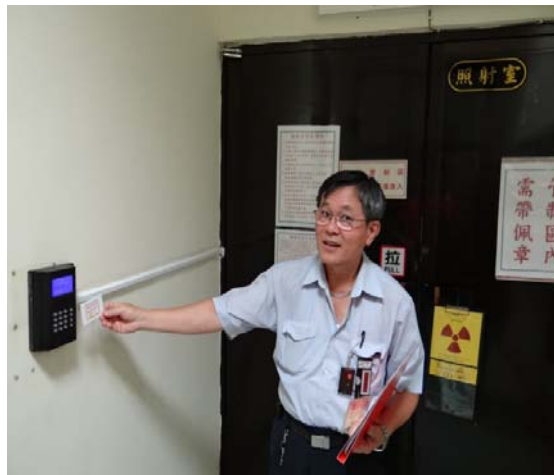
Figure 1. Access Control–Swipe card reader to control personal entrance and exit
