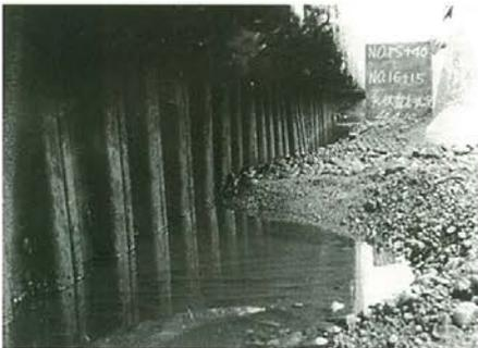
Seawall basement bared by beach erosion
