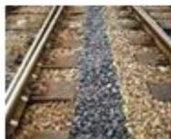
**Lateral End Restraint for S&C/Curves**
