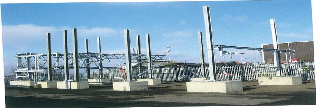
Figure 11: Mock-up of overhead line installation for training technical staff on the new equipment.
