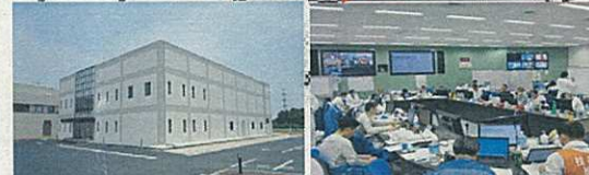
Seismic Isolated Building Emergency Response facility with seismic isolated structure
