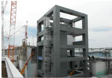
Completed fifth section of framework Photograph taken on April 10, 2013
