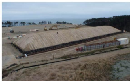
Condition of 1 st facility (photographed on March 27)
