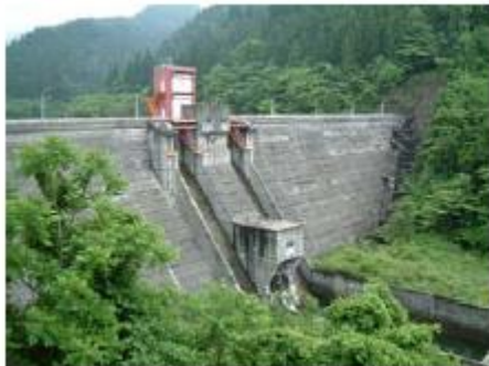
Photo 4. Tobe Dam(改建前)
