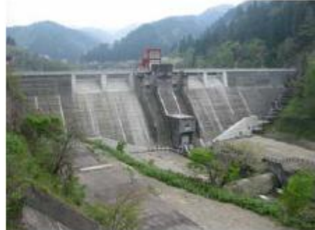
Photo 5. Tobe Dam(改建後)
