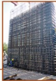
Iron reinforcing bar assembly of wall foundation
