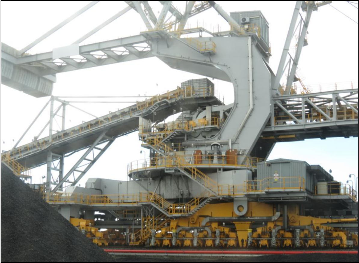
圖81 NCIG 斗輪式堆/取煤機(Bucket Wheel Stacker/Reclaimer)局部
