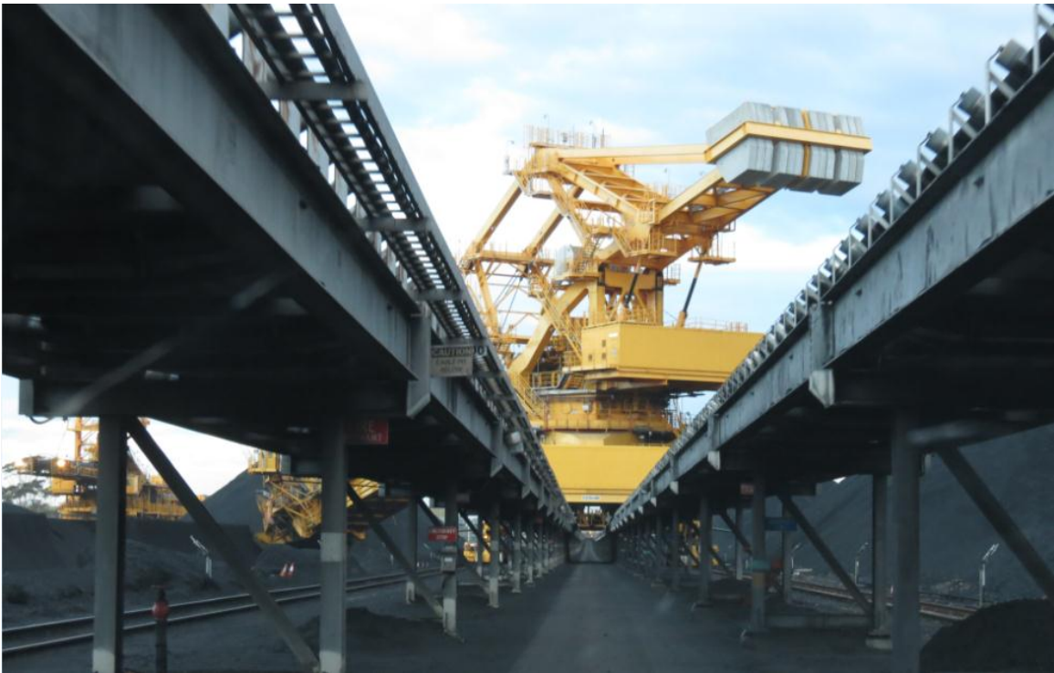
圖62 PWCS 斗輪式堆/取煤機(Bucket Wheel Stacker/Reclaimer)取煤作業
