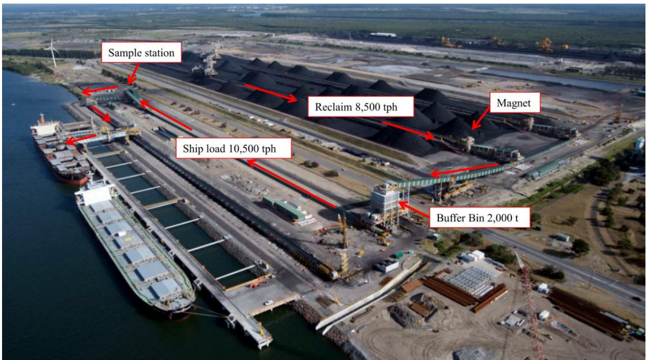
圖92 NCIG Shiploading System
