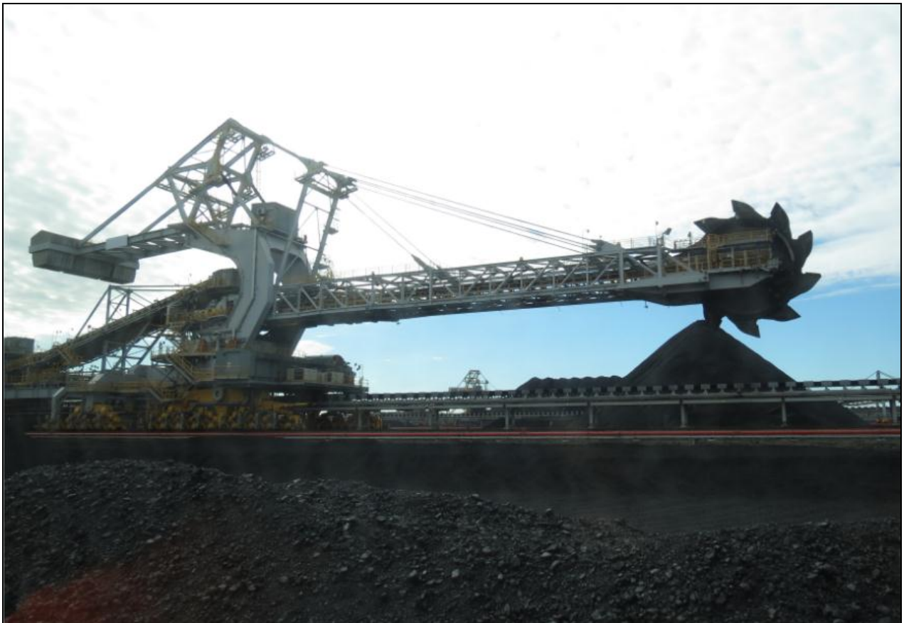
圖80 NCIG 斗輪式堆/取煤機(Bucket Wheel Stacker/Reclaimer)
