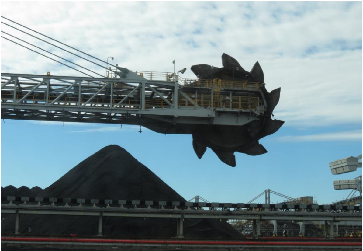
圖82 NCIG 斗輪式堆/取煤機(Bucket Wheel Stacker/Reclaimer)局部
