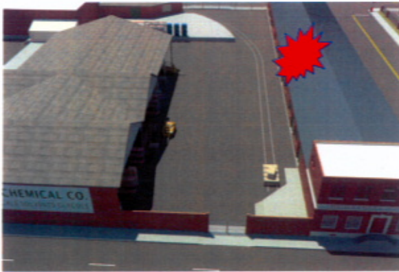
Open shed storage area
