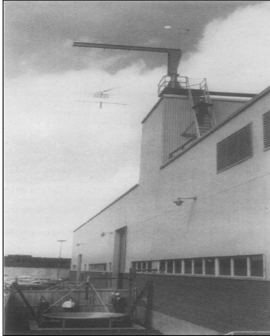
Figure 4. Experiment for microwave-powered helicopter (From [7]).
