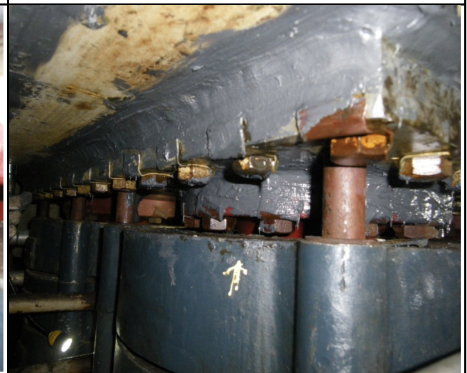
High Voltage Bushings AB膠塗佈
