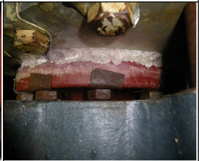
High Voltage Bushings 塑鋼土修補
