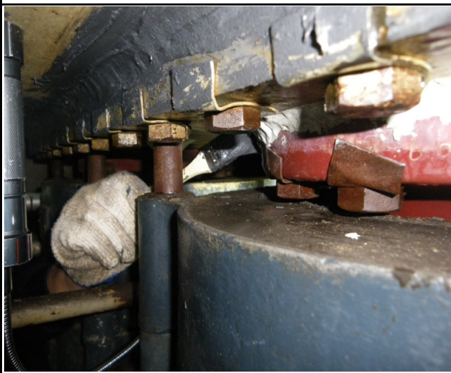
High Voltage Bushings AB膠塗佈
