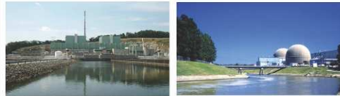
The Surry Power Station (right) is a Westinghouse pressurized water reactor (PWR) design with a large, dry subatmospheric containment and is located in Surry, VA.
