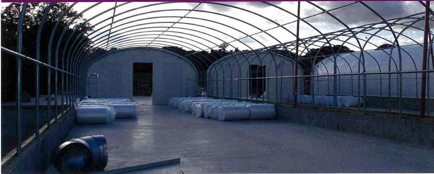
JFM sheds being constructed.
