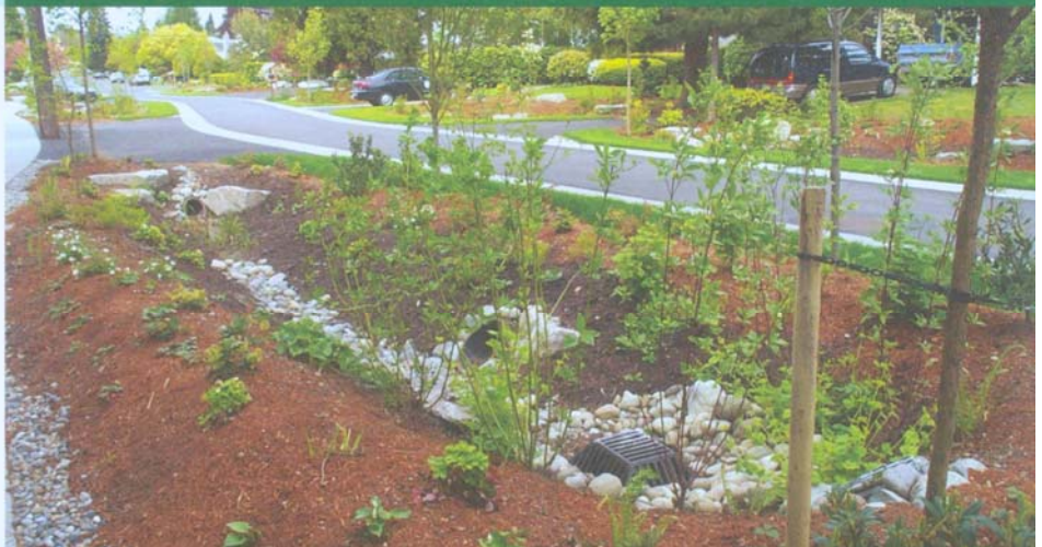
Infiltration swales along the first SEA Street
