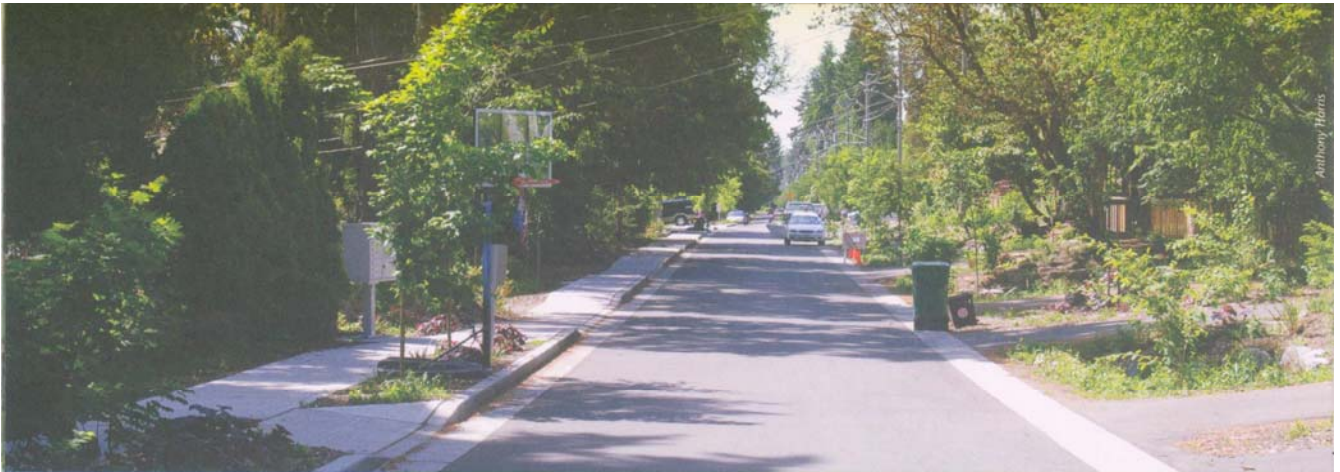
The Pinehurst NDS locates large, deep swales on one side of the roadway
