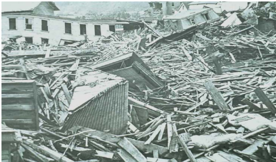
South Fork 壩潰壩後下游災損情形
