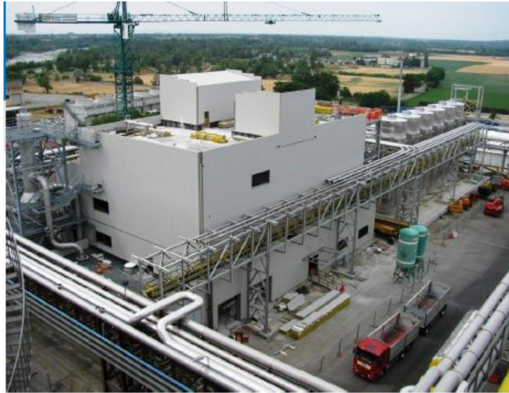
World's 1 st commercial bio-succinic acid plant Cassano, Italy; start-up Q4-2012
