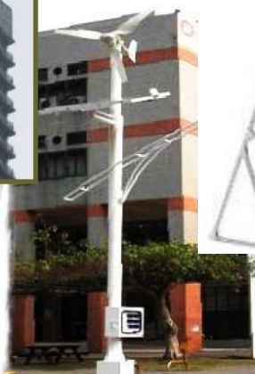
Sin Ta Wind-Solar hybrid system
