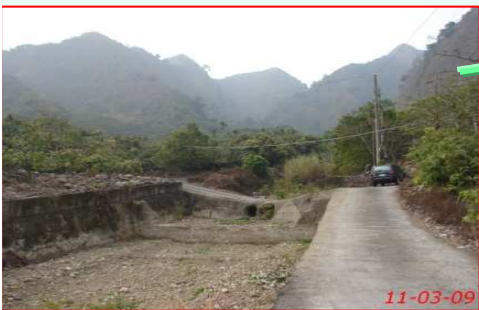
Overflow point at begin of opening
