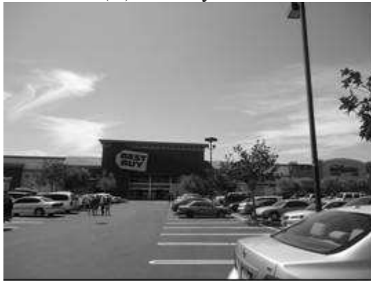
(C) Downey Landing Retail Center
