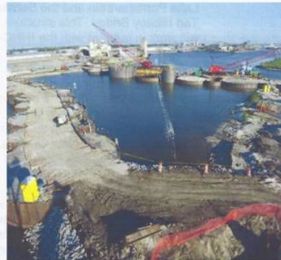
North and south cofferdam walls
