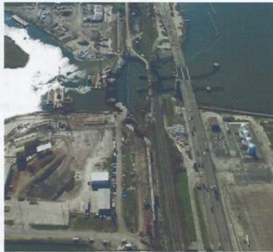
Aerial of Seabrook Floodgate Complex
