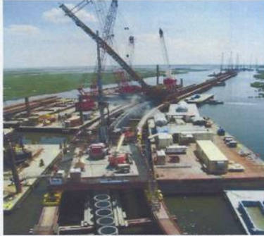
Construction of the barrier wall
