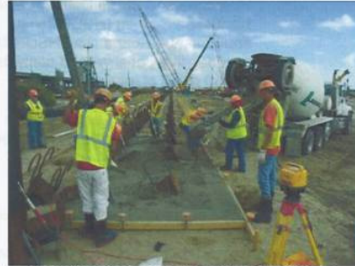
Construction of western floodwall tie-in
