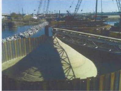
Coffer cell sand fill operation
