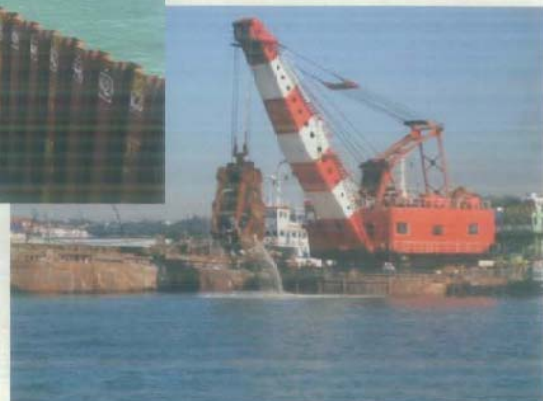
Dredging by Grab Dredger
