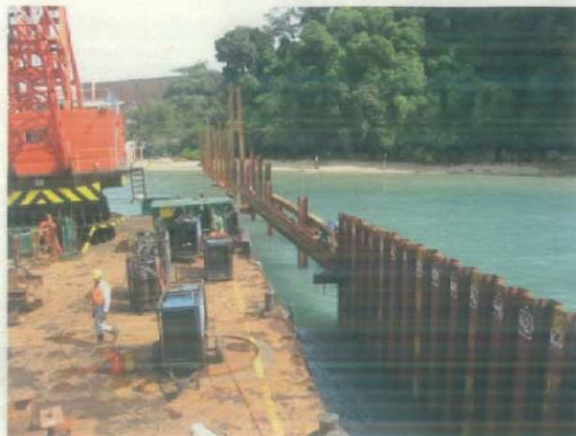
Cofferdam Installation
