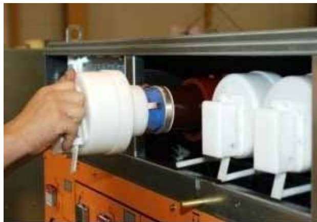
簡潔/緊密箱型開關 (Compact Package Switchgear)
