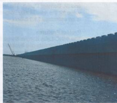
Flood side of the barrier wall
