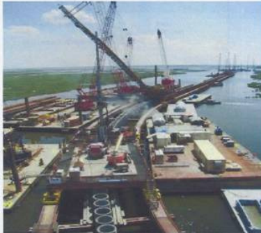
Construction of the barrier wall
