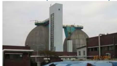
蛋形消化槽(7000m 3 /槽)x2顆
