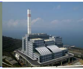
Resource recovery plant/modern incinerator
