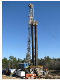
Rig on location at well D9-8#2
