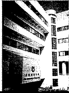
Use of architectural design in form of cantilever floors for providing sun shades
