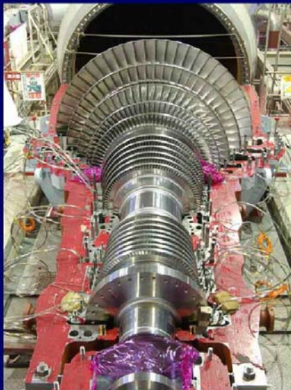
Special Measurement (LOWER CASING & ROTOR INSTALLATION)
