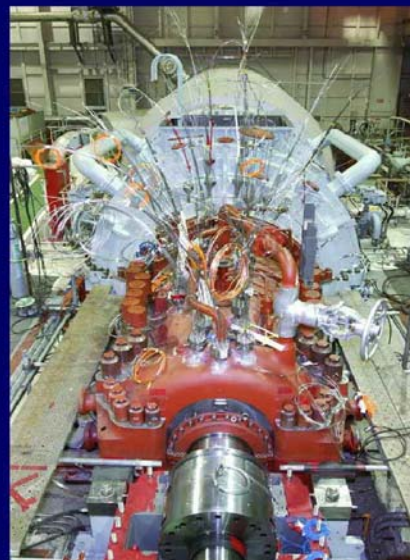
Special Measurement (UPPER CASING INSTALLATION)
