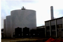
The slurry remains in the reactor for 15 to 20 days to form a stable post-fermentation digestate material
