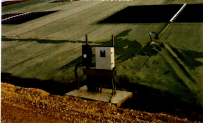
Facing the right direction, geomembrane sideslopes on which the solar panels are mounted have an angle of approximately 18 degrees from horizontal
