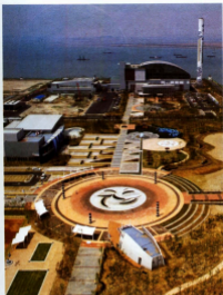
A Waste to Energy facility in Incheon, South Korea - a country which has progressively adopted forward-thinking European limits
