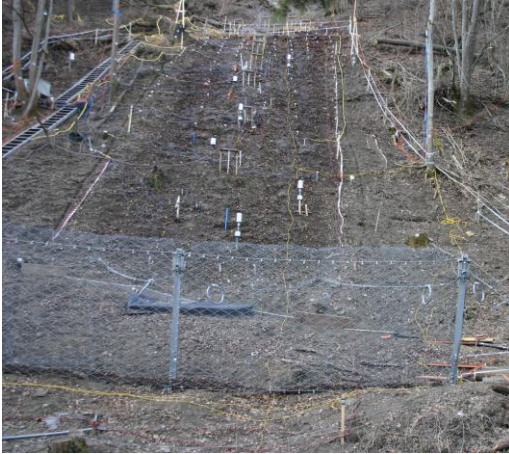
Instrumented slope in Rüdlingen, SH.
