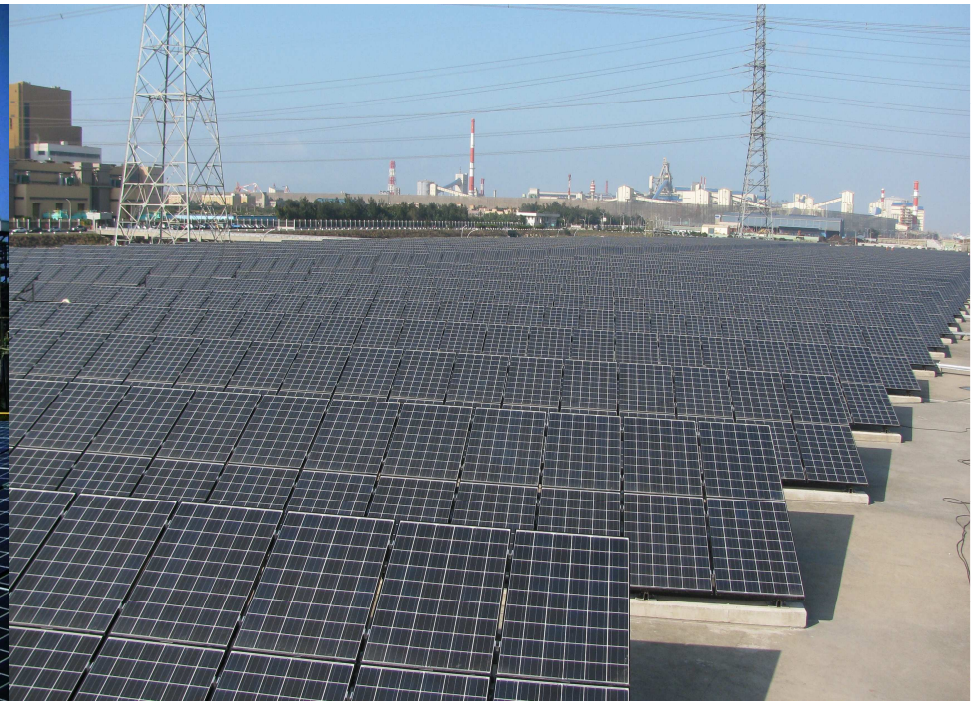
Raw Water Tank, Taichung Power Plant 1.5MW
