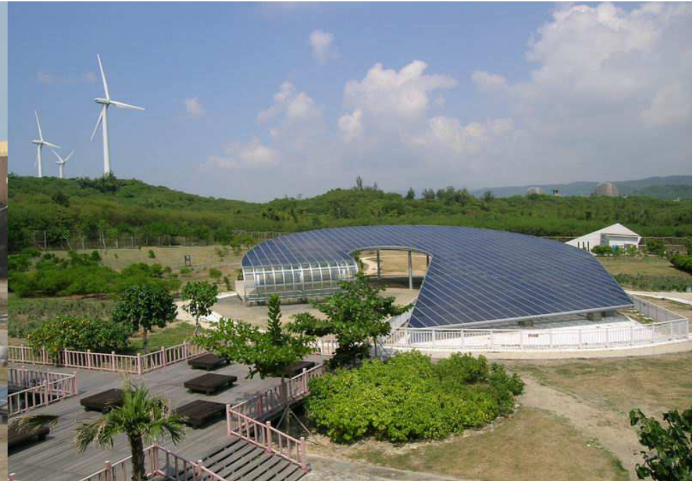
South Visitor Center near the 3rd Nuclear Power Plant 50kW
