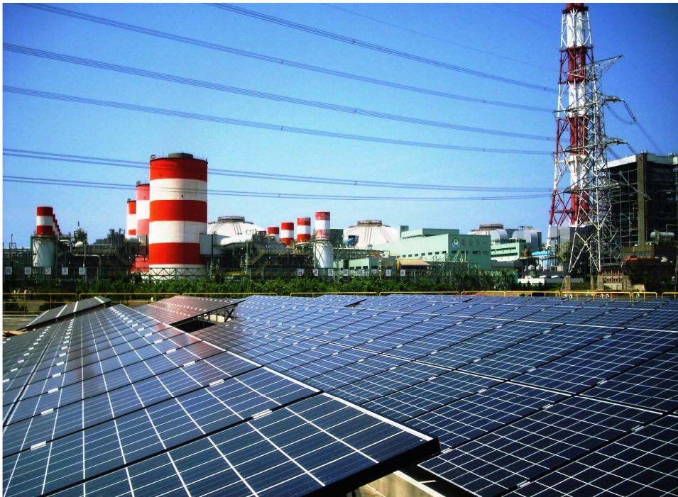
Raw Water Tank, Hsinta Power Plant 1.0MW
