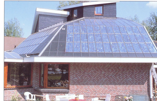
Plate 9 Energy-autonomous house at Woubrugge, The Netherlands (Ecofys) BOALsolar profile system
