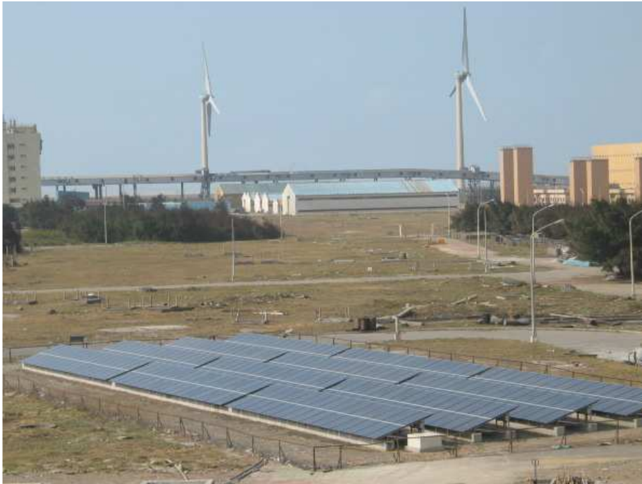
Taichung Power Plant 72kW
