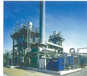
Submerged combustion furnace High-temperature oxidation furnace for high-COD waste liquids
