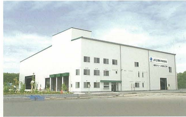
Yokohama Clean Resource Recycling Plant
