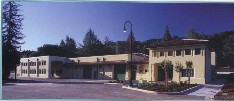
The Orinda Water Treatment Plant treats water for more than half of EBMUD's customers.
