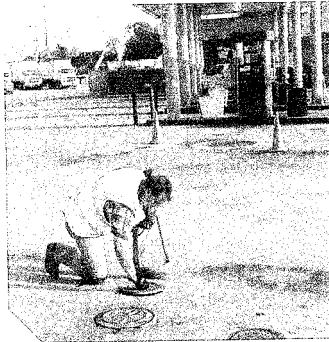
Inspecting a spill bucket
