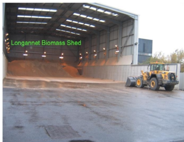
圖七、Biomass storage shed
