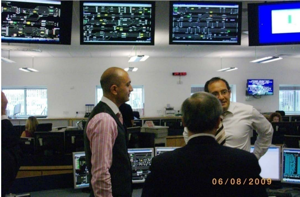
照19. 參訪Network Rail Integrated Control Centre
