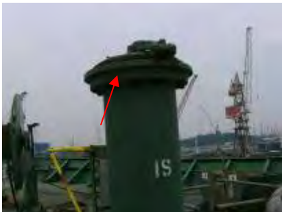
1s 艙 gas free cover 修理
