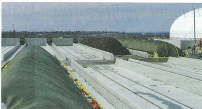
The material is then trucked and placed on a concrete pad, in long rows called windrows. The GORE cover, a specially developed membrane laminated between two polyester layers, is pulled over the material and secured to the ground.
