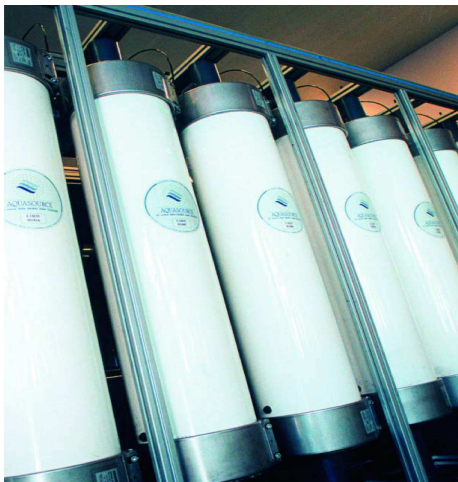
Aquasource Modules in a Rack
