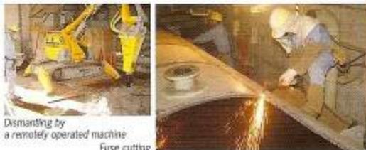
Dismantling by a remotely operated machine
