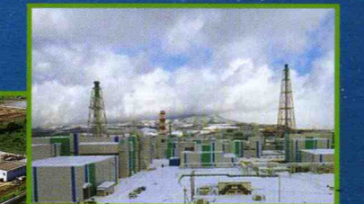
Reprocessing Plant (Rokkasho Mura) (Photo: Courtesy of Japan Nuclear Fuel Limited)
