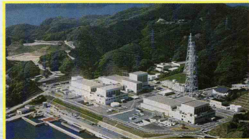
Tohoku Electric Power Co., Inc. Onagawa Nuclear Power Station
