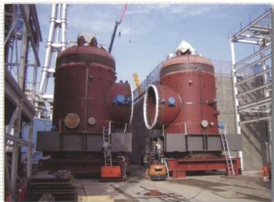
〈Pressure Vessel Components for Gasifier and Syngas Cooler〉
