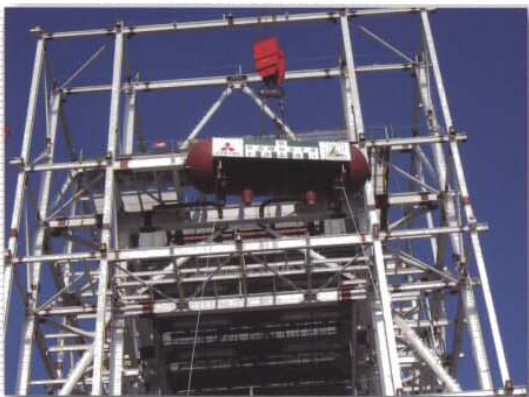
〈Steam Drum Lifting for HRSG〉
