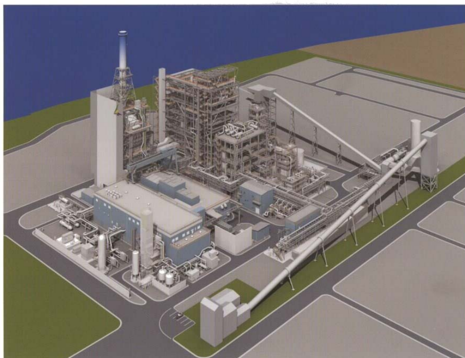
Bird's-eye view of IGCC Demonstration Plant
