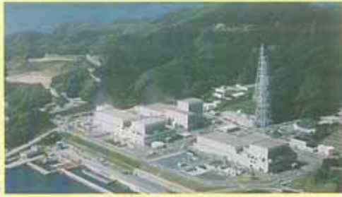
Tohoku Electric Power Co., Inc. Onagawa Nuclear Power Station
