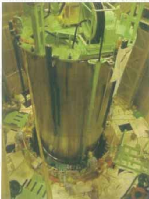
Replacement of Shroud
