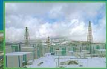
Reprocessing Plant (Rokkasho Mura) (Photo: Courtesy of Japan Nuclear Fuel Limited)
