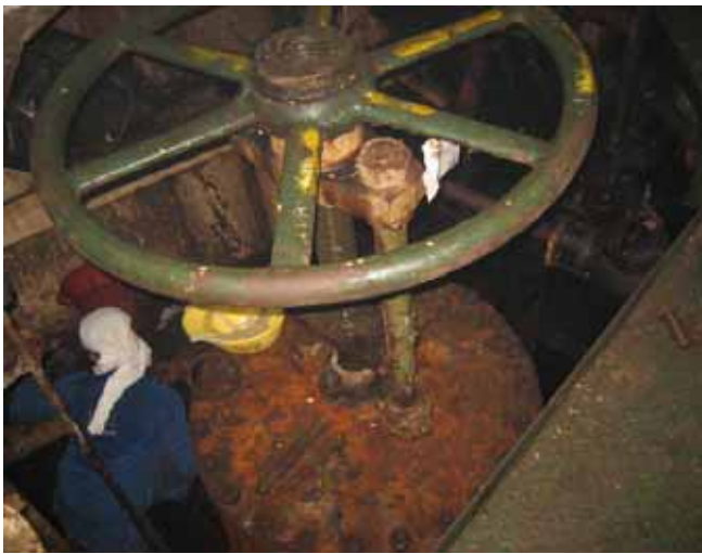
OVERBOARD SEA VALVE 安裝
