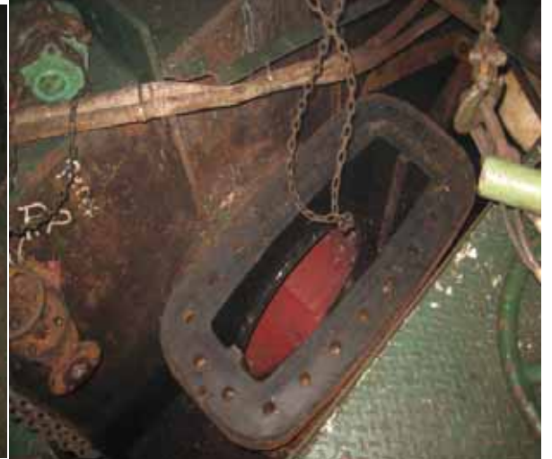
OVERBOARD SEA VALVE 安裝
