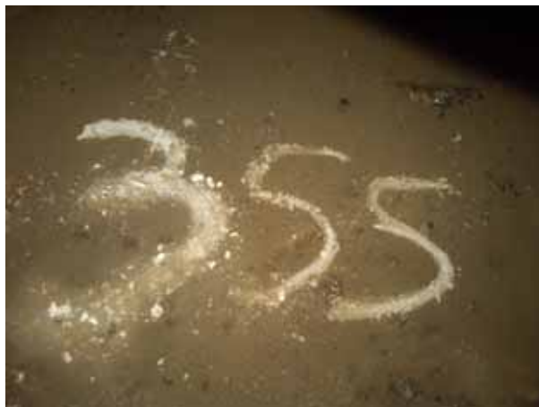
Bellmouth No.3S stripping
